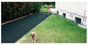
The cells of the grid can be filled with soil and seeded to have a driveable grass area or filled with gravel or decorative stones. The holes between each of the cells of the grid, promoting better growth of grass. Unsightly ruts, mud and pot-holes are eliminated. Storm water seeps back into the ground rather than running into drainage systems.
